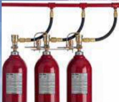
Carbon dioxide fire suppression system
