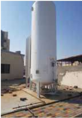
LPG vertical tank with evaporator
