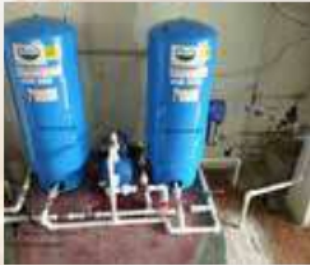
Installed water pump with pressure tank
