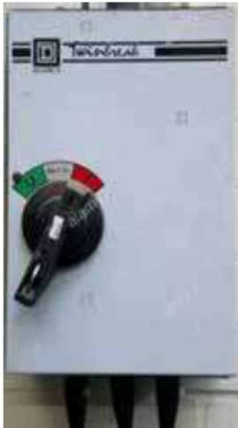
Industrial Enclosure with breaker enclosure
