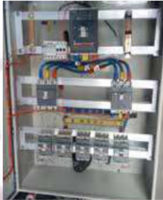
Main Distribution panel Board
