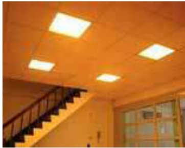
False ceiling mounted LED 60 X 60 Light
